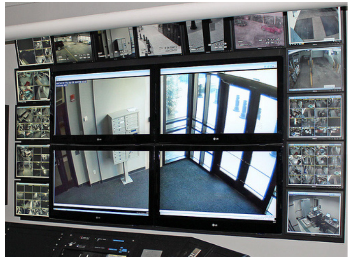
Guards view the exacqVision VMS software in the command center on seven 42-inch LCD monitors and 15 19-inch monitors.
